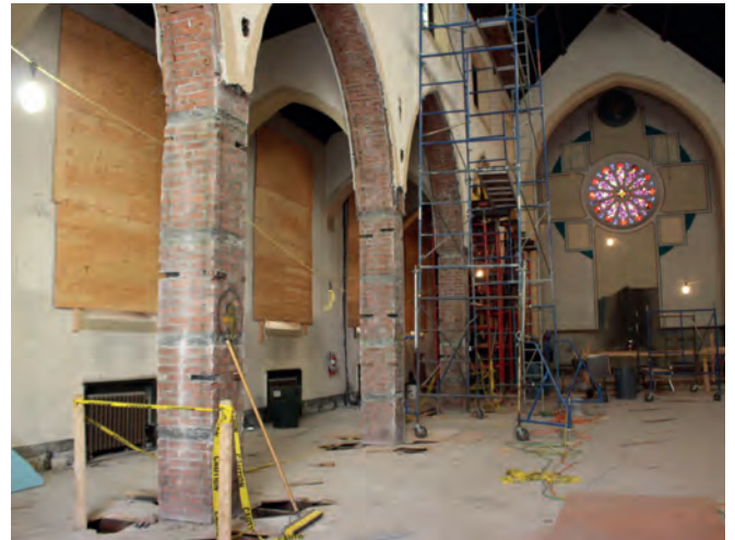
Renovation work underway 2014
